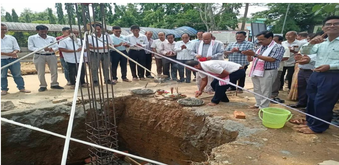
Started construction of College Main Gate on 07-06-2024
