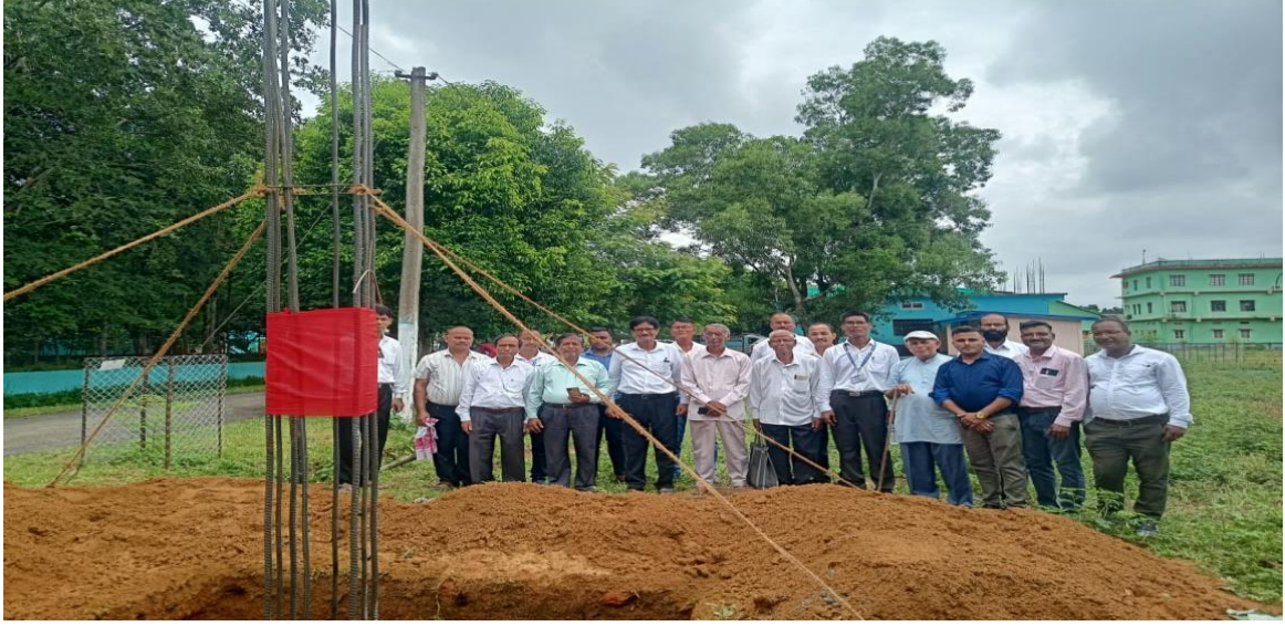
Started construction of SATIRTHA BHAVAN on 03.08.2023
